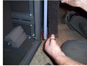
2. Lightly pull the foam taut to the bottom bracket
